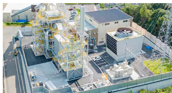
Minokamo Biomass Power Plant
